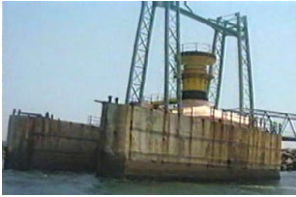
Fig. 1. Indian wave power converter (OWC) [15]
