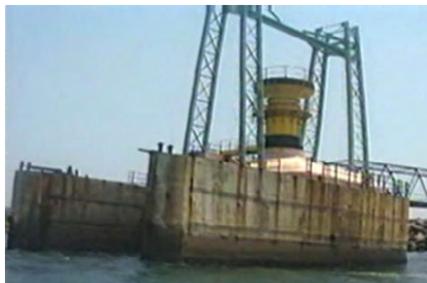
Fig. 1. Indian wave power converter (OWC) [40]
